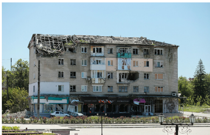
Fig. 3 Damage to residential homes and businesses in Izium city.
