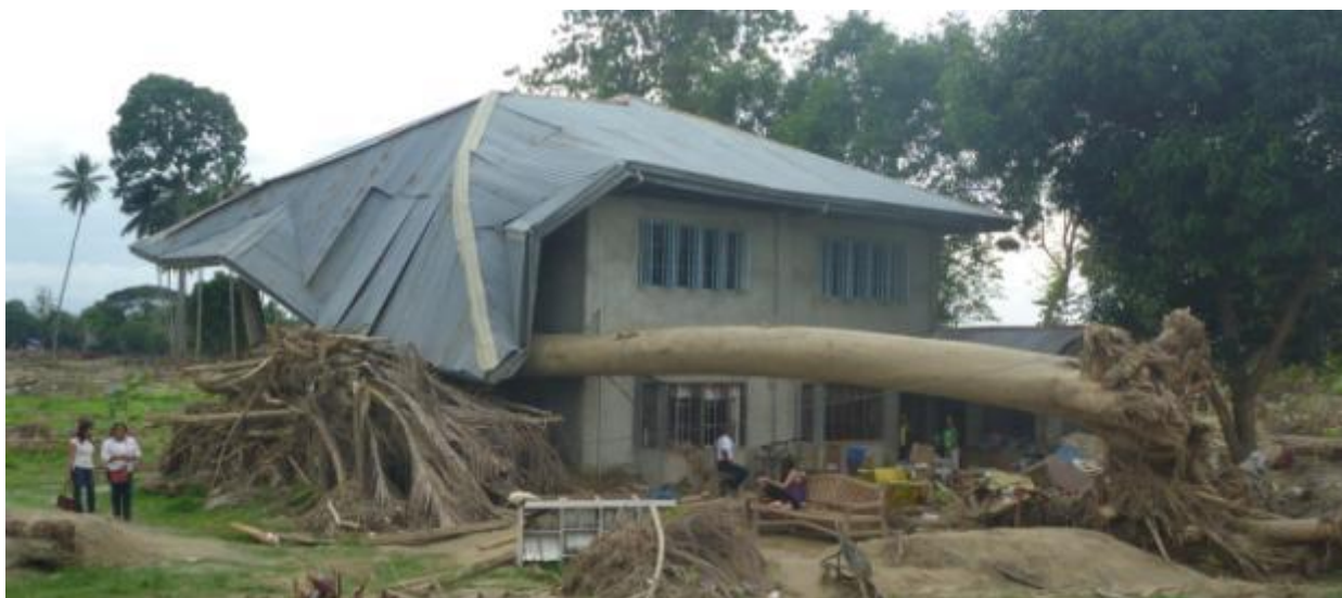
A house partially damaged by a falling tree in Bayug Island Iligan where 2,500 people are displaced.
