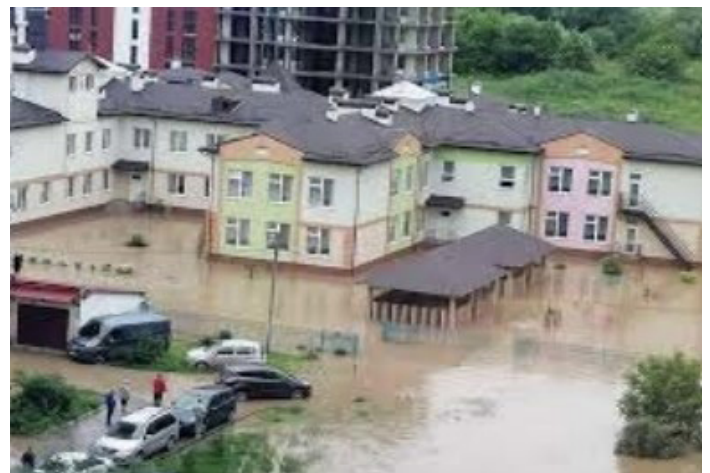
Image 1. Photo of flooded houses during the 2020 Western Ukraine floods. Source: IFRC. 17
