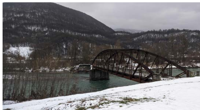
Image 3. Collapsed bridge in Tiachivska, Zakarpatska oblast, due to flooding.
