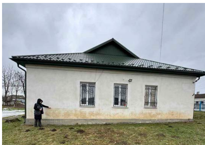
Image 2. Flood level visible at on a home in Halytska, Ivano-Frankivska oblast.
