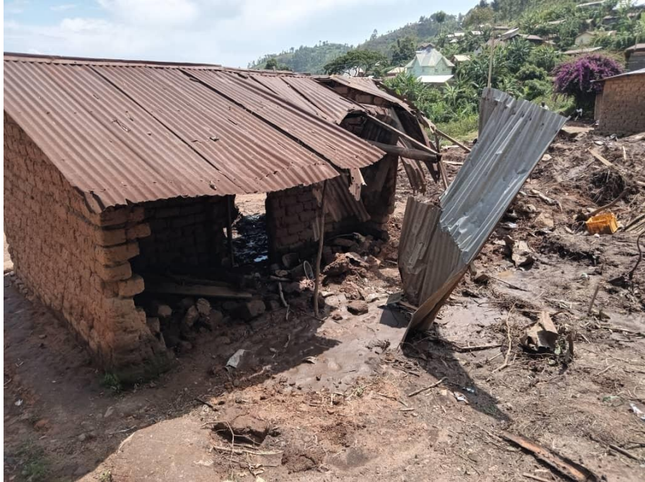
Shelter destroyed in the territory of Kalehe, South Kivu
