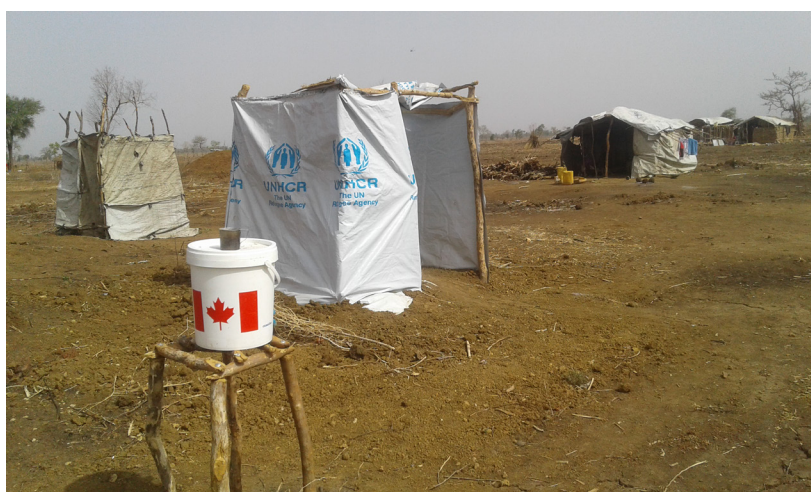
Figure 3: Household latrine with plastic sheet and hand-washing facility in Doro camp extension site
