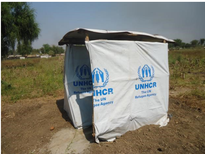
Figure 1: PSN latrine with wider entrance built in concrete
