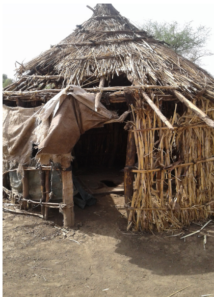
Figure 2: Household latrine built with local materials
