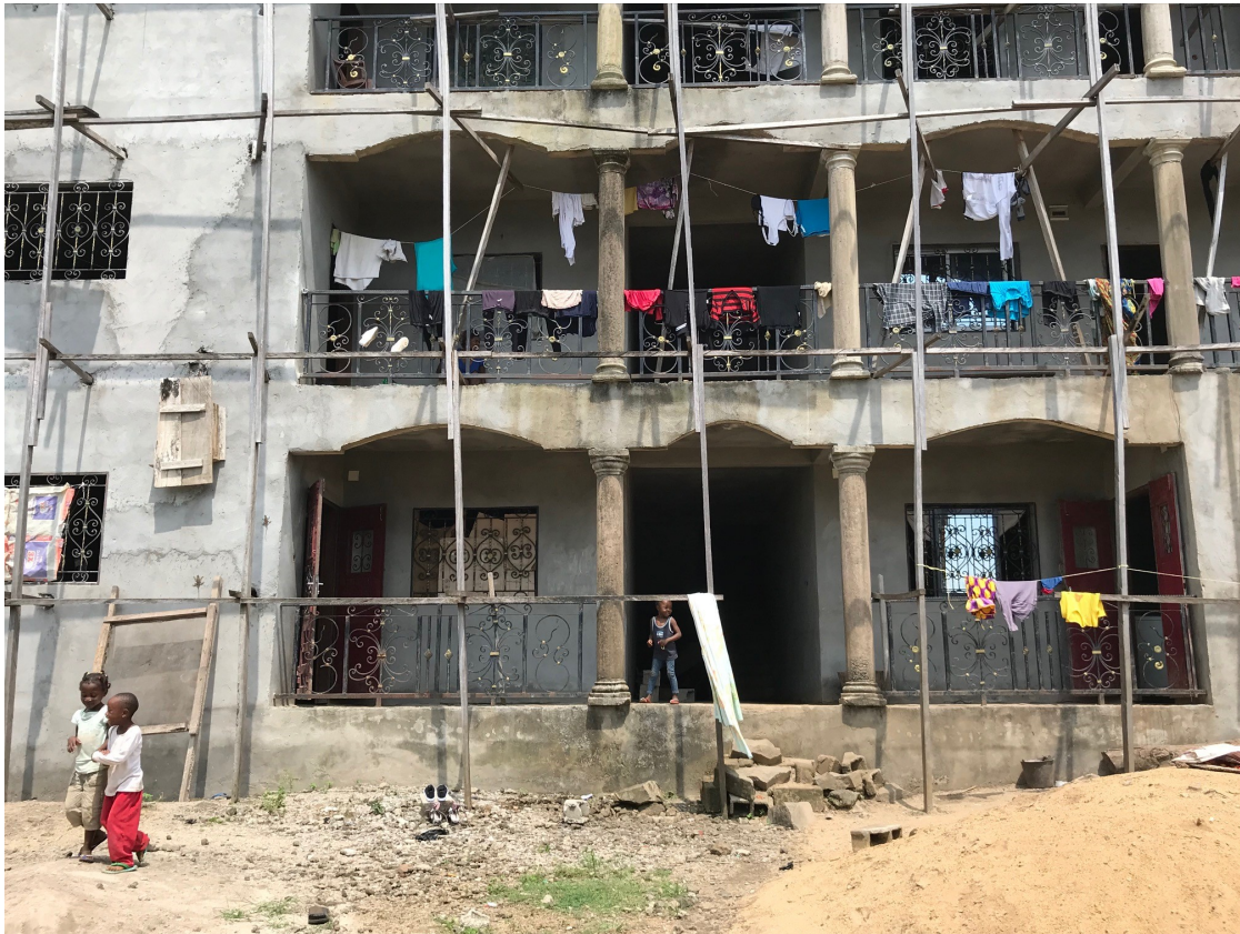
Unfinished buildings, Lime area, Cameroon, 2018. Cameroon's Shelter Cluster Team.
