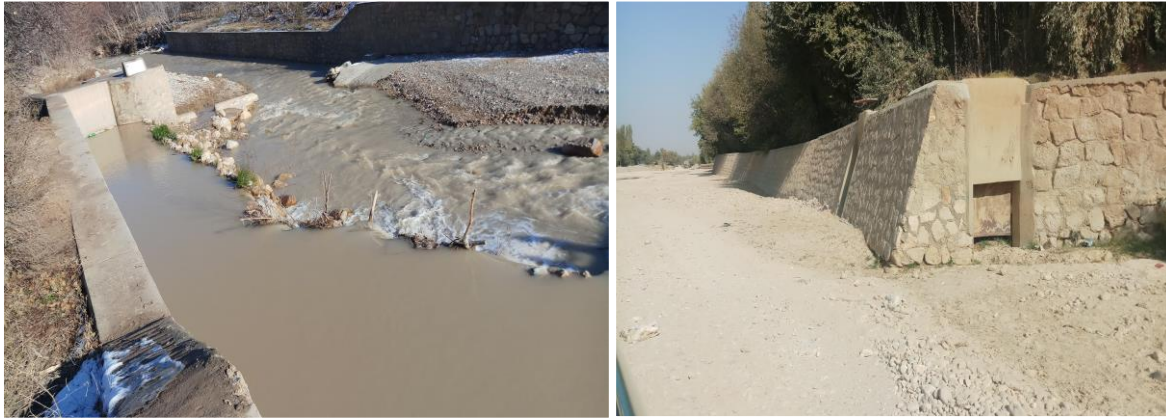
Photo 1: Photographs of abgardan (left) and gate (right) in Khulm District. Photo Credit: Kandiwal Wali, December 2020.
