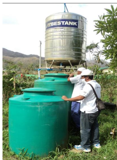
Figure 14: Slow sand filtration water system in rural areas
