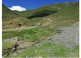
Water pipeline and rock-falls
