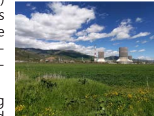
Hrazdan Termal Power Plant
