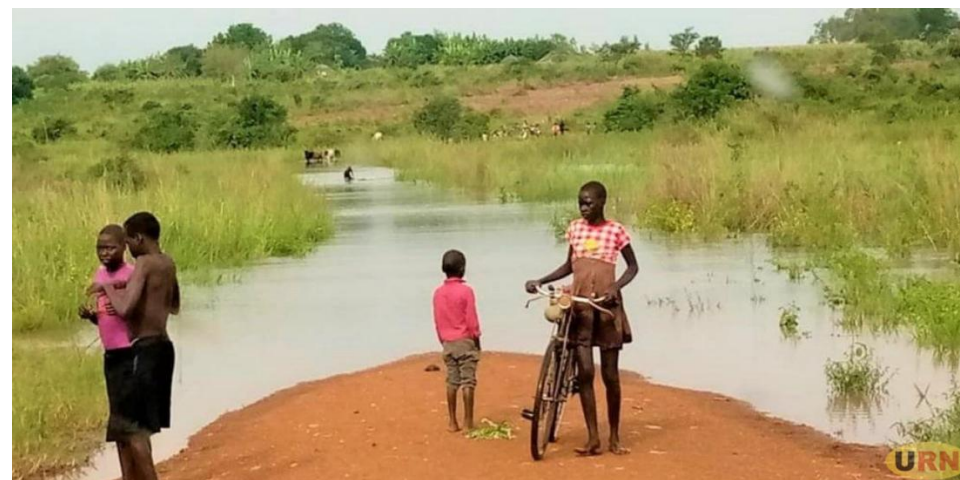
Photo 2: A section of the road that has been completely submerged in the flood water in Mucwini East Subcounty Kitgum District. Photo Credit: URN
