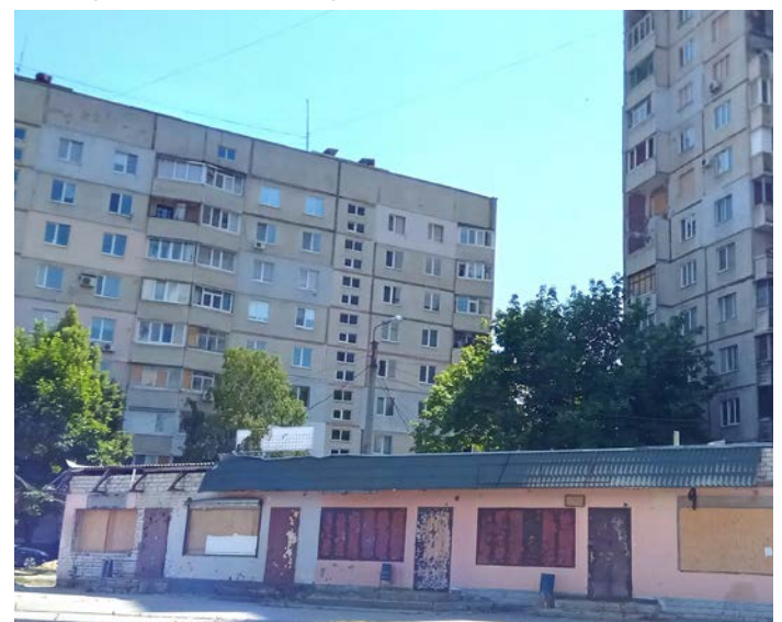
Image 3: Damaged public infrastructure in Kharkiv, July 2024 (REACH field team)
