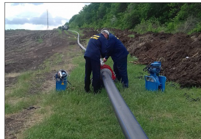
Repair works on the water supply system in Volnovakha Raion, 31.07.2020. By Voda Donbass Company.
