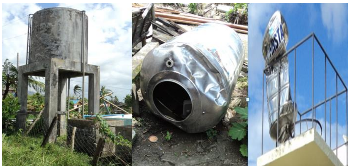
Figure 11: Undamaged masonry water tower (left). Damaged tower metal tanks (centre, right)
