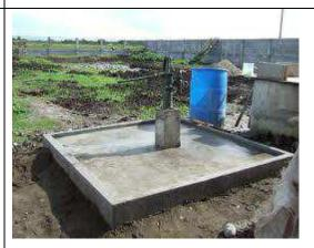
HAND PUMP. Surrounding area is protected by RC slab. No cracks, no infiltration by surface water
