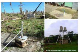
Water supply system common in rural areas. Gravity system or connected to an elevated tank with the following basic scheme: well/spring – pump –transmission pipe-elevated tank – distribution pipe to community taps
