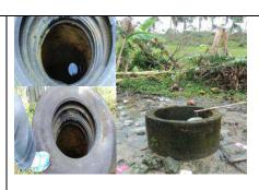
Walls are not lined or partially lines. No RC slab and spill way is present. Easy pollution from surface
