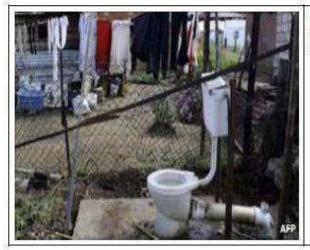
Flush toilet, separation of excreta from human contact guarantee, involved technology foresees piped water and septic tank or sewerage system.
