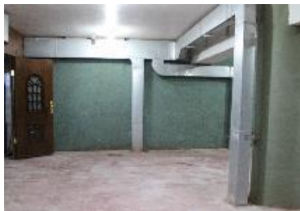
Figure 33. Water tank installed in the building above the alternative underground hospital
