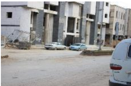
Figure 14. External perimeter of the building above the alternative underground hospital (before protective wall was built)
