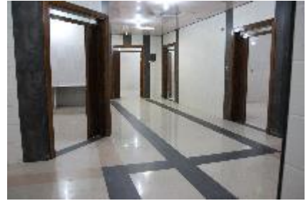
Figure 24. Alternative underground hospital facilities after tiling had been completed
