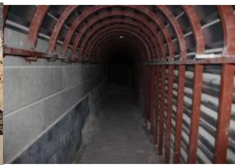
Figure 18. Inside view of exit tunnel 1
