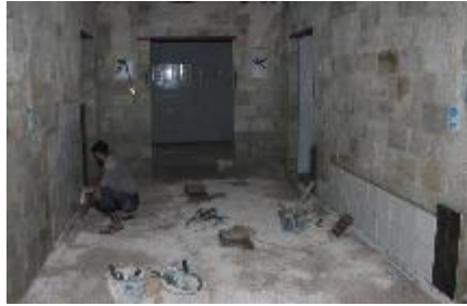
Figure 23. Plastering and tiling of walls and floors
