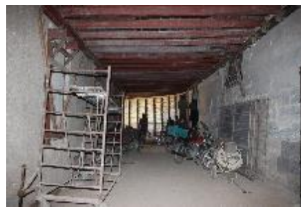
Figure 21. Inside view of exit tunnel 2
