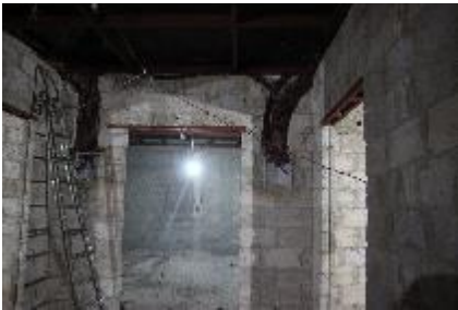
Figure 25. Overview of the electrical conduits installed
