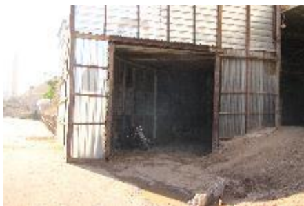
Figure 20. Front view of exit tunnel 2
