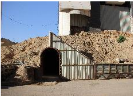
Figure 17. Front view of exit tunnel 1
