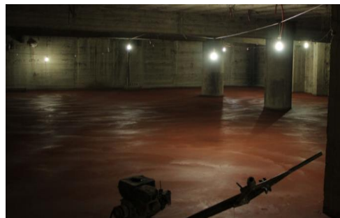
Figure 5. Second floor of basement after completion of slab
