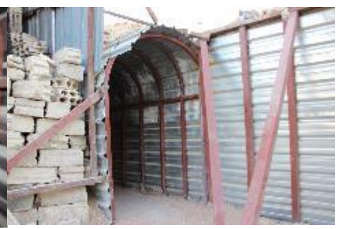
Figure 19. Behind view of exit tunnel 1
