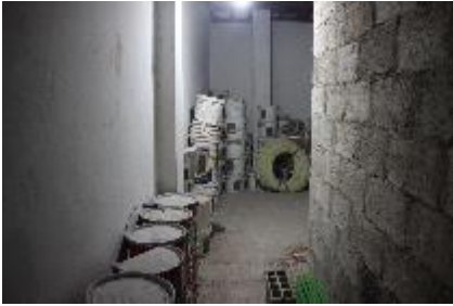
Figure 22. Storage of materials to be used for hospital rehabilitation
