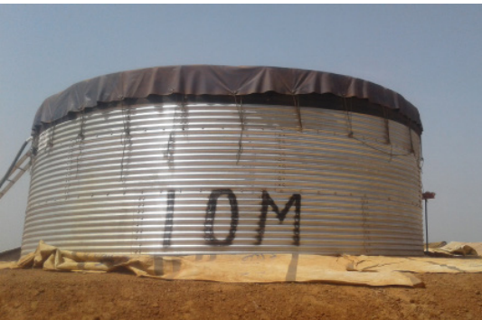
Figure 1: Water tank supplying water to two sectors of the PoC
