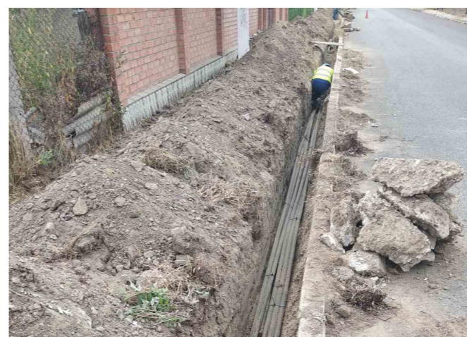
Underground power cables under repair, 09.09.2020
