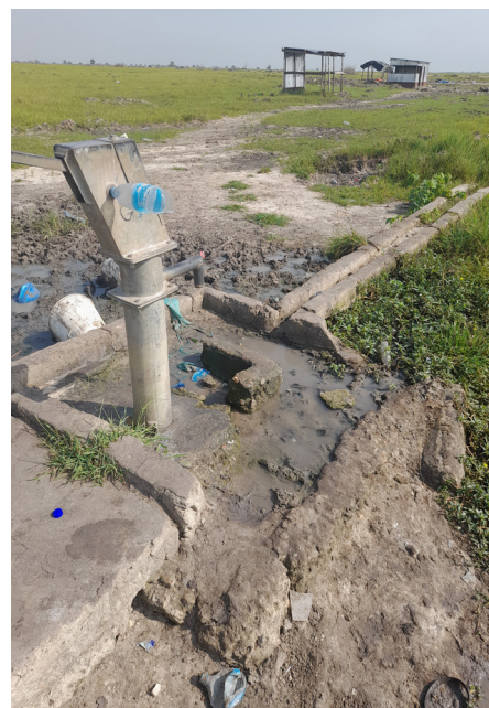
Functional borehole in Kongor Payam without proper apron; June 2026
