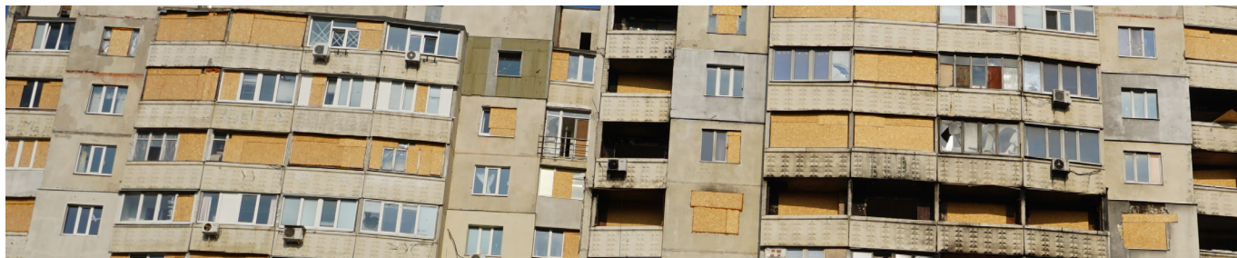
Image 3: Wooden panels covering windows to protect them from damage during shelling. Source: REACH.
