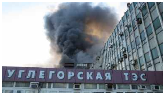
Vuglehiska TPS damaged by shelling, 27.07.2015 By RBC.ua
