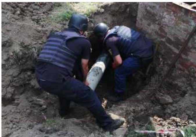
Detection of an explosive object in Myronivske, on the territory of Myronivska heating power plant (HPP), 03.08.2018 By SESU
